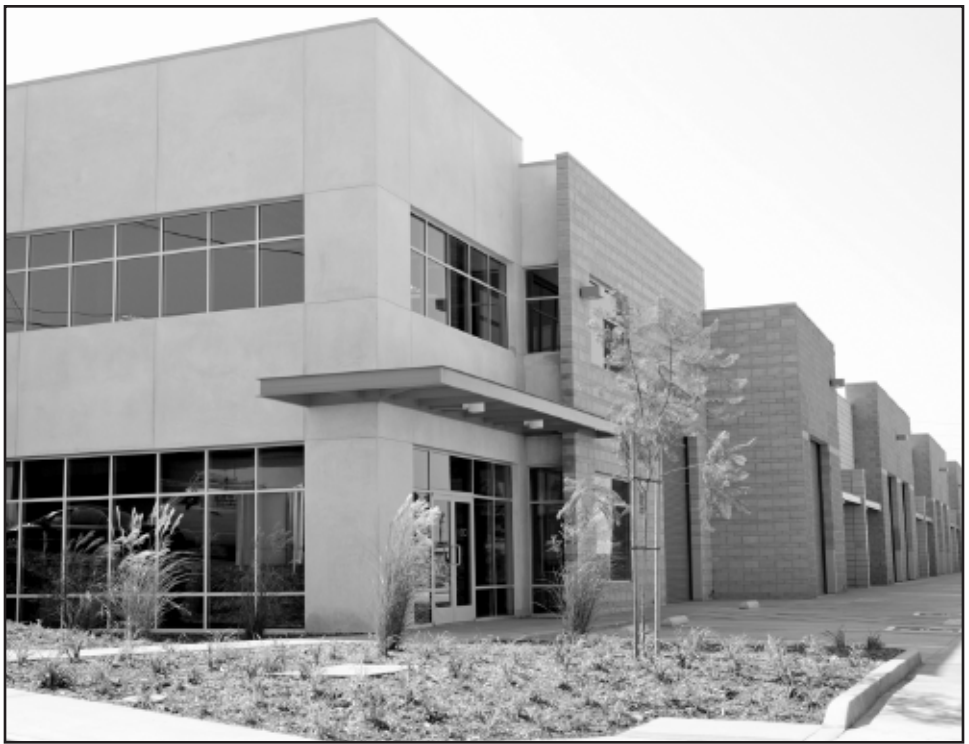
A 28,000-square-foot development by B.J.H. Leasing Inc. at 2445 Palm Dr. recently completed. The industrial facility includes nine suites, 14-foot loading doors, 18-foot interior clearance, skylights and 46 parking spaces. Howard CDM oversaw construction, and Withee Malcom Architects designed the facility. (Photograph by the Business Journal's Thomas McConville)
