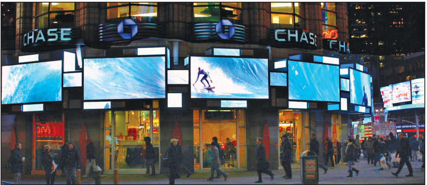
Quicksilver's 12-by-100-foot digital display spans across the retail store's facade at nighttime at the corner of Broadway and 42nd Street. Today's digital displays include cameras that support interactive functions for passersby. (TDI Signs photograph)
