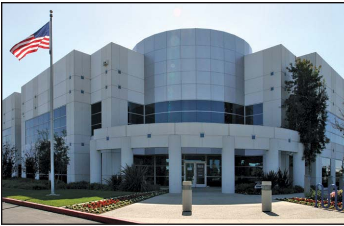
Watson Land Company leased a near 150,000 square foot industrial property to Herbalife International Inc. at 18431 Wilmington Ave. within the master-planned Dominguez Technology Center. The company relocated its operations from its previous 82,000-square-foot location within Watson Industrial Center in Carson. (Photograph by Watson Land.)
