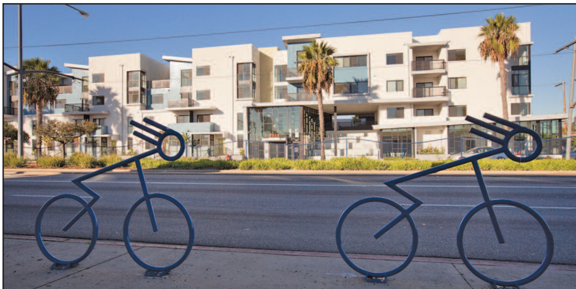
The Long Beach and Burnett Apartments is a 46-unit, mixed-income, multi-family housing development at 2355 Long Beach Blvd. in Central Long Beach. The Blue Line connecting Downtown Long Beach with Downtown Los Angeles passes by the project. (Photograph by the Business Journal's Thomas McConville)
