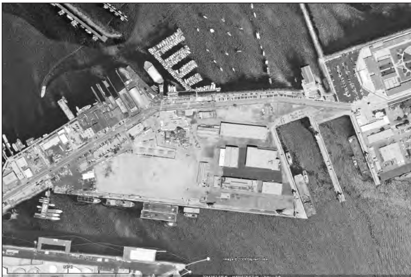
An aerial view of the Southwest Marine Berth 240Z at the Port of Los Angeles shows the two deep-water slips that Gambol Industries hopes to use as a dry dock to service ships 650 feet and smaller. Gambol has projected that revitalizing the site as a working shipyard with heavy-duty electric cranes could generate 1,000 jobs. The Los Angeles City Council has ordered port officials to study the idea. (Photograph courtesy of Gambol Industries.)
