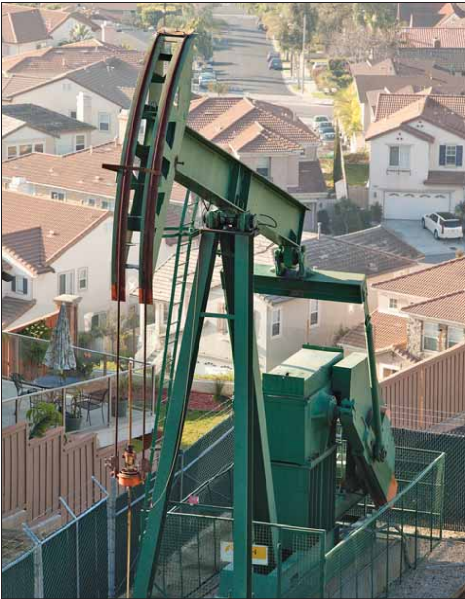
Oil pumping stations are located throughout the City of Signal Hill as the city and developers have worked around the oil wells, developing homes and commercial businesses. (Photograph by the Business Journal's Thomas McConville)
